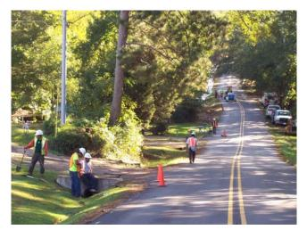
with trying to determine the best way to replace over 40,000 linear feet of sewer line, in a timely, economically feasible manner without overly disrupting the general public. Guest Consultants, Inc. proposed pipe bursting as a method of pipe replacement instead of the traditional pipe laying method involving extensive excavation and disturbance. This method not only saved on excavation expense, but also minimized damage to streets and was also much less disruptive to the traffic.
